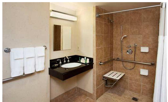
Figure 7: ADA compliant bathroom in a traditional hotel. Note grab bars and roll-in shower stall.
